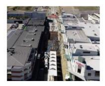
Last month the hours of work in Hibberson Street were extended in an effort to fast track completion of various activities such as rail stop build, track slab and rail install, pole and overhead wire install. Works have progressed very well to the point where the intention now is to...
